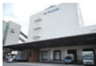
Jonanjima plant of KYOKUYO AKITSU REIZO CO., LTD.
