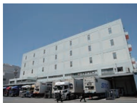
Tokyo plant of KYOKUYO AKITSU REIZO CO., LTD.
