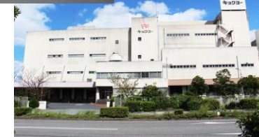
Fukuoka cold storage facility
