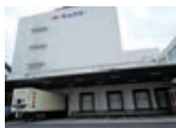
Jonanjima plant of KYOKUYO AKITSU REIZO CO., LTD.
