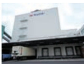
Jonanjima plant of KYOKUYO AKITSU REIZO CO., LTD.
