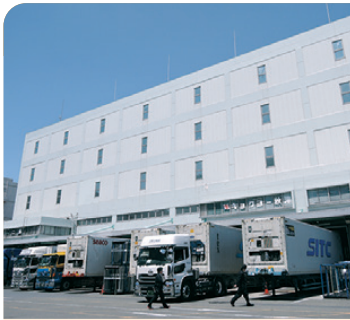
Tokyo plant of KYOKUYO AKITSU REIZO CO., LTD.
