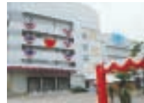
An external view of the plant
